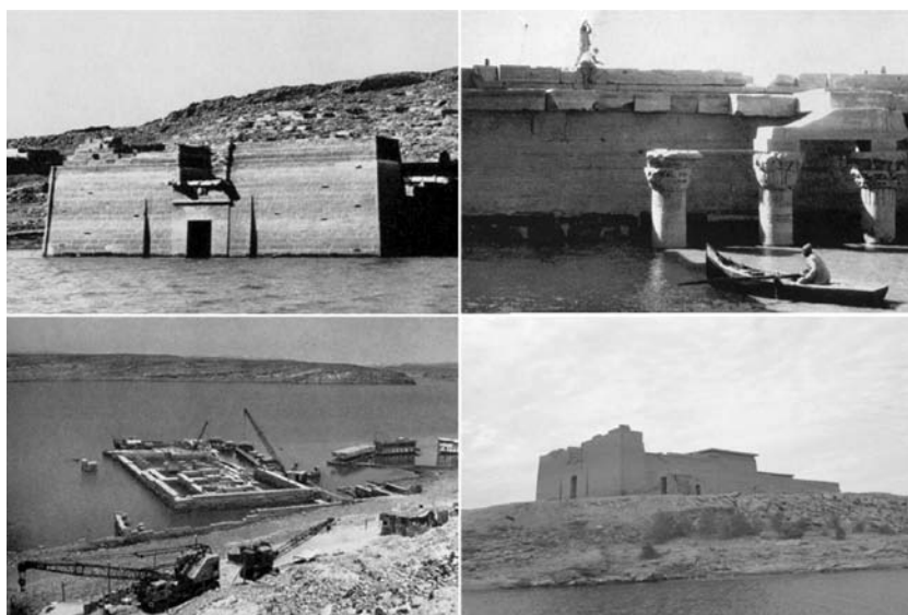
Fig. 2. The dismantling and reconstruction process [Wright 1972].
